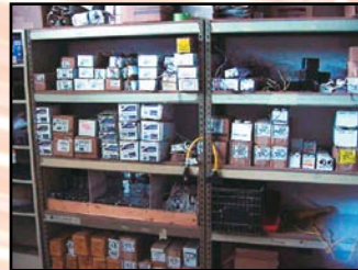
VIEW OF BALLASTS
