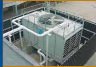
BAC CHILLING TOWER
