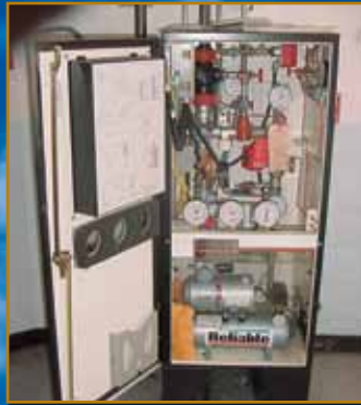
RELIABLE SELF-CONTAINED FIRE SPRINKLER SYSTEM
