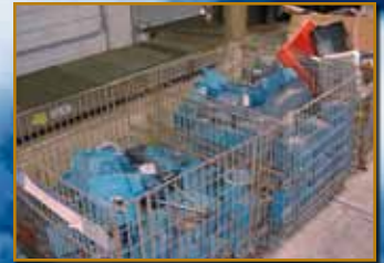
VIEW OF CONVEYOR DRIVE MOTORS
