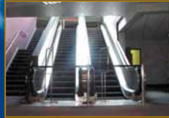
VIEW OF ESCALATORS
