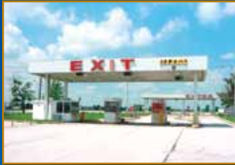
PARKING CANOPY W/CASHIER BOOTHS
