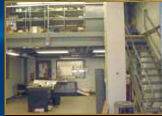
VIEW OF STEEL MEZZANINE
